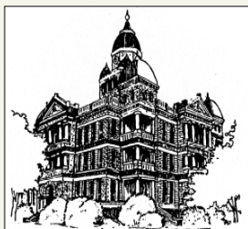
1896- Denton County Courthouse-
